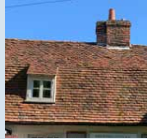
Plain tile and red brick chimney stack
